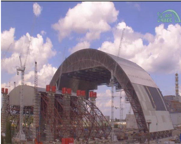
Photo: Construction Site of the Chernobyl NPP as of May 29, 2014
