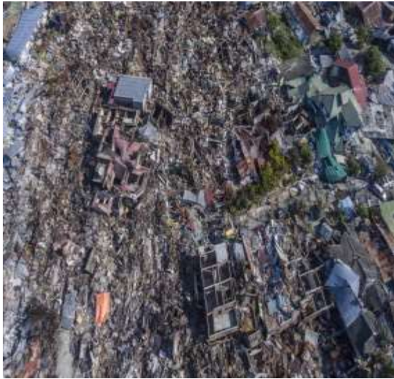
Photo: Liquefaction impact, Palu, Indonesia, www.bbc.com
